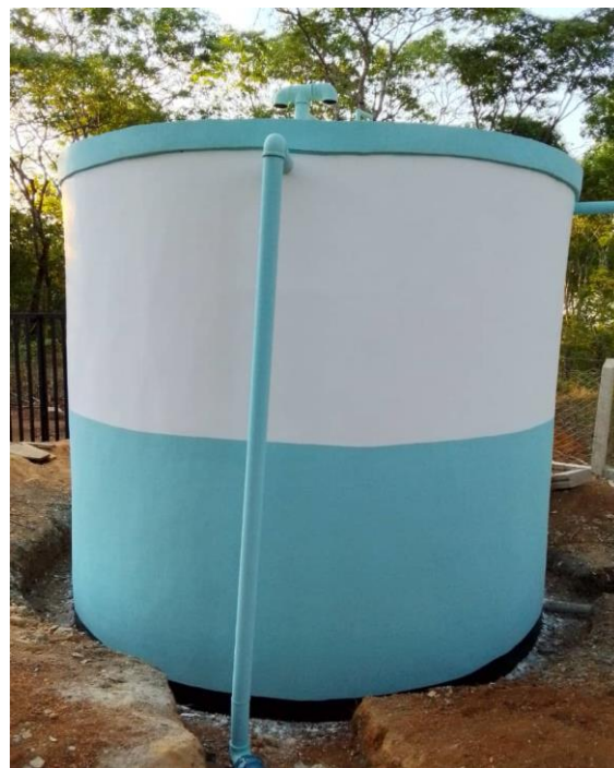
One of the fenced Break Pressure Tank constructed
