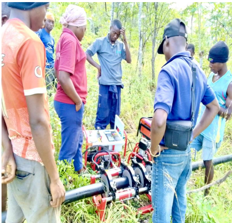
Fixing and joining water pipes by fusion
