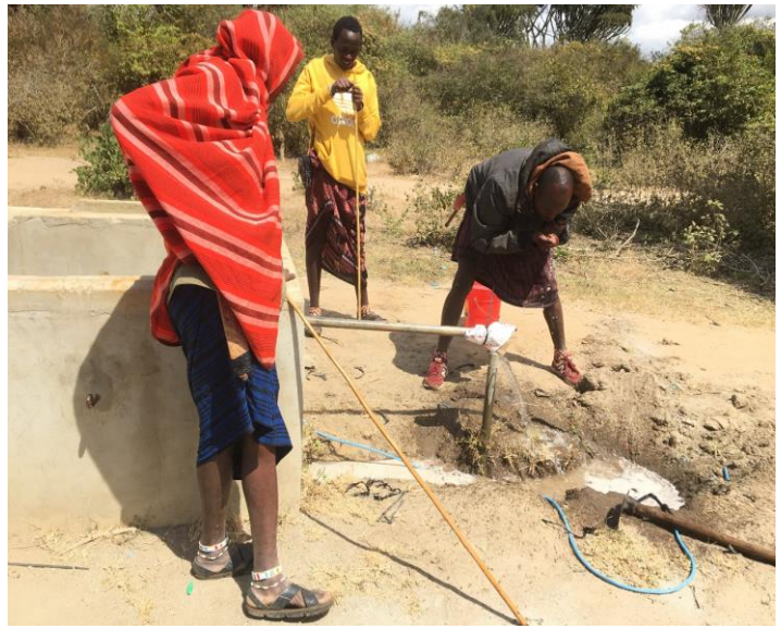
Testing after maintenance – Ilikandururo WSP
